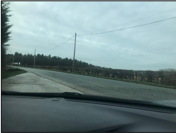
Mill Lane access looking west
